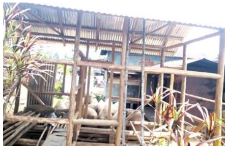
Plate 20: Wooden frame of Khasi house.
