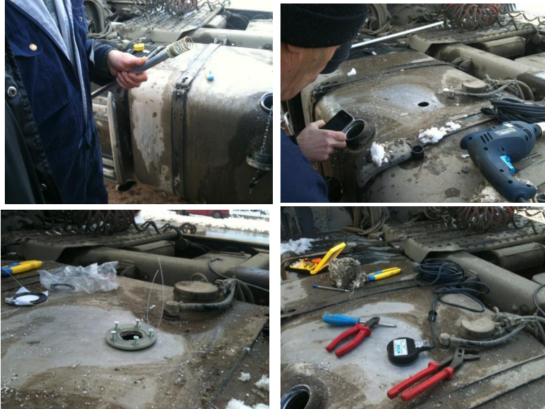
Fig. 3. Procedures for fitting the sensor to the tank
